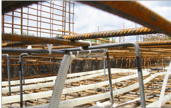
View into concrete ceiling under construction with integrated cooling pipes (left) and geothermal pipes (right) before placement in the ground. Source: Fraunhofer ISE.
