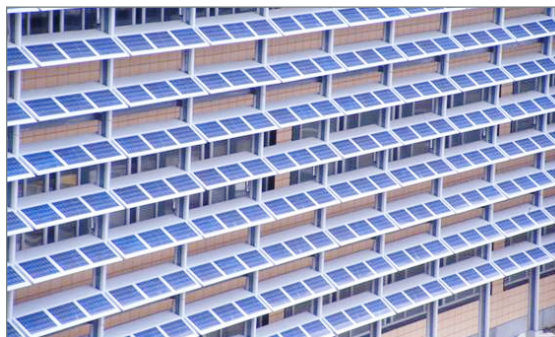
Sun shades produce electricity while providing passive solar shading. Source: ECN / Bear Architects, Netherlands.
