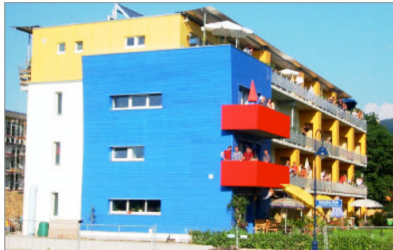
One of thousands erected in central Europe, the solar passive house (top) uses thick insulation and triple-glazed windows to keep annual heating loads below 15 kWh/m 2 . This building is equipped with a newly designed compact heating and ventilation device (left) that integrates solar thermal collection, earth heat exchanger, heat pump, and heat recovery systems to efficiently provide domestic hot water, space heating, and ventilation. Source: Fraunhofer ISE.
